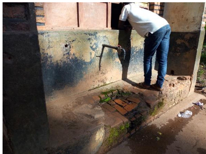
Photo: @Biryogo Water Station
