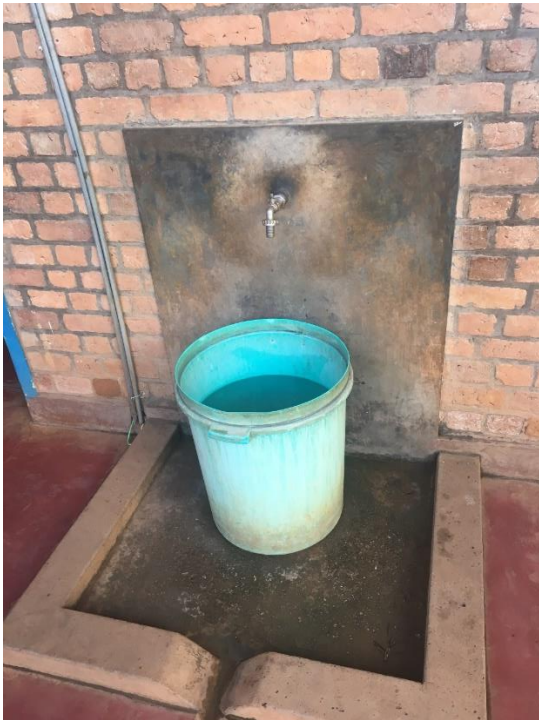
Photo: @ Handwashing facilities in rural area (Gasabo)
