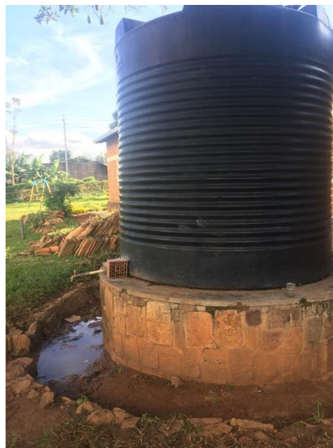
Photo: @ A water tank in Humura Centre
